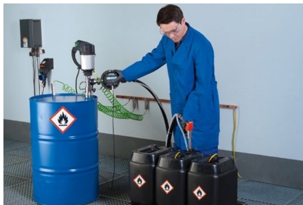
Semi-automatic canister filling in Ex-zone 1.
