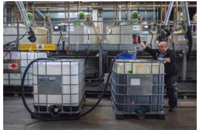
F 430 being used to pump out of an IBC.
