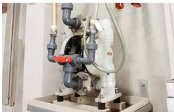
FDM: pumping nickel chemicals to prepare an electroplating tank.
