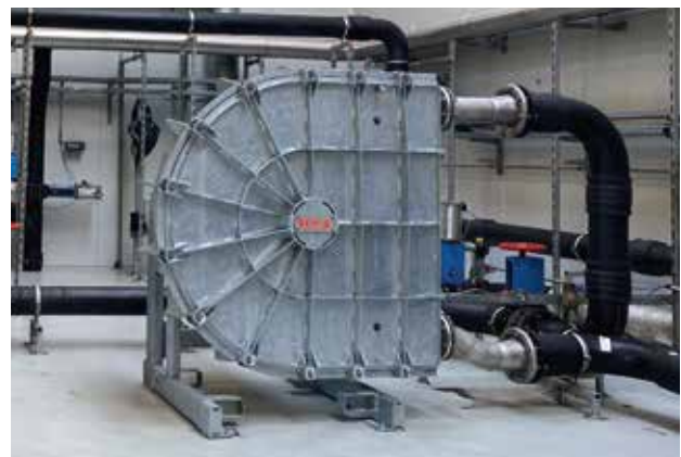
pumping wastewater containing solids: the PERIPOWER achieves displacement volumes of up to 300 m 3 3/h.
