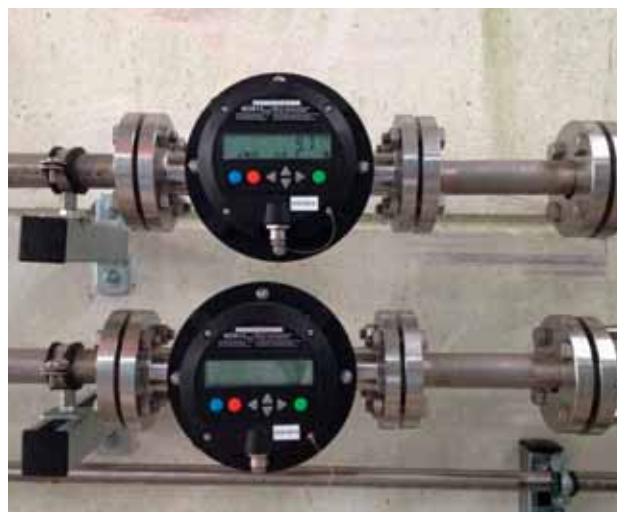
FMO 150 with flange connection installed in a pipeline.
